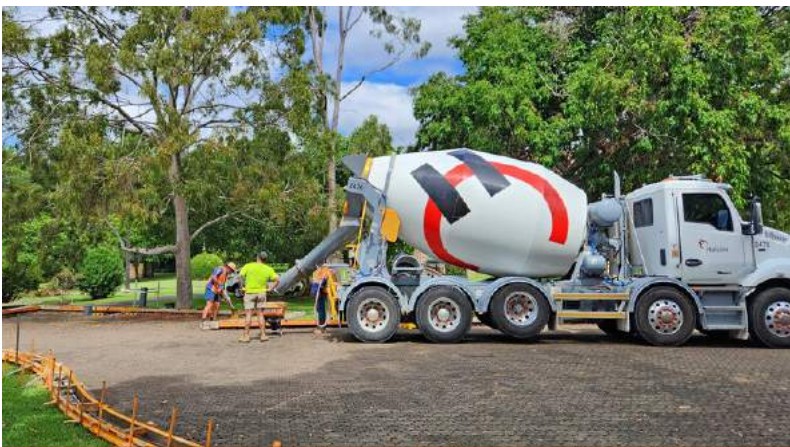
Montbel: repairing edges at parking area.
