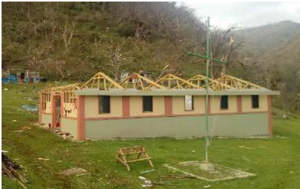
Area council building
