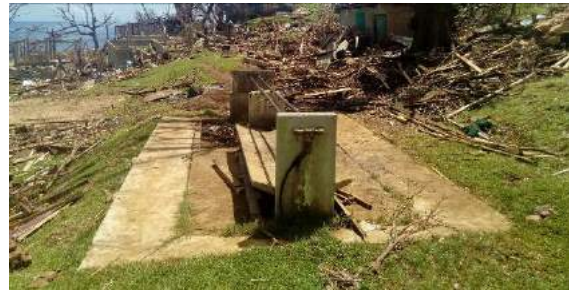
Non-functional public water taps
