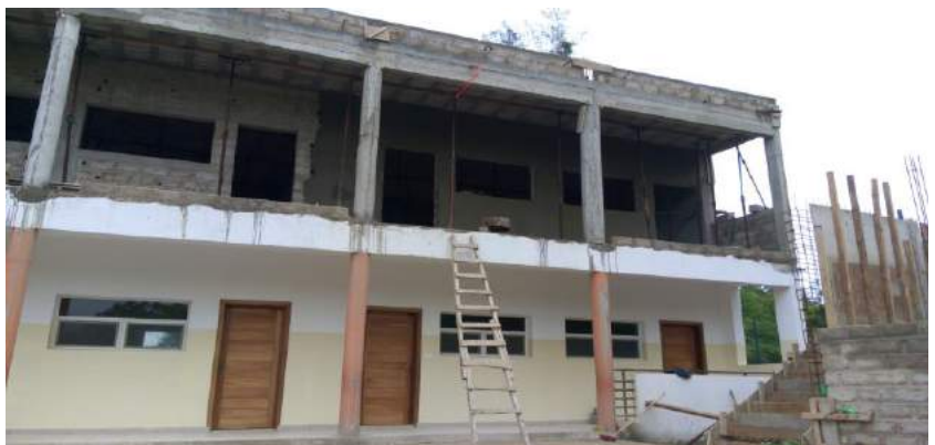
Work continuing in the new class rooms (bloc A)
