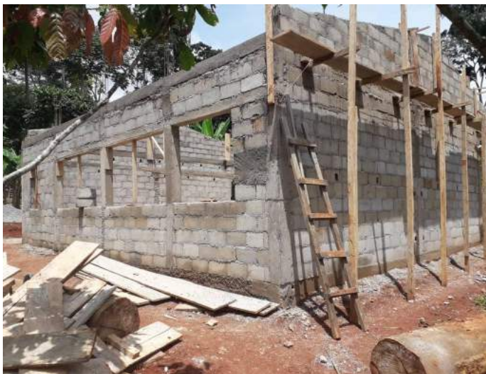
The Italian foundation "Meoni" funded the construction of a classroom at the Marist Center for Ecological Agriculture. Then a road was built. This eases access to the site.
