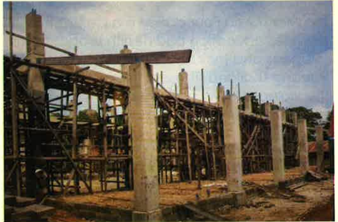
Above: Church under construction
