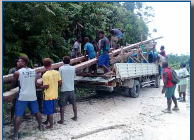
Above: The men have their teams for the next stage of carting the timber to the building site.
