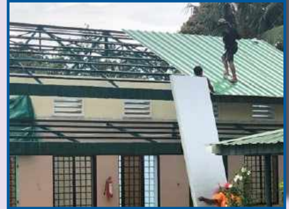
Above: New Roofing
