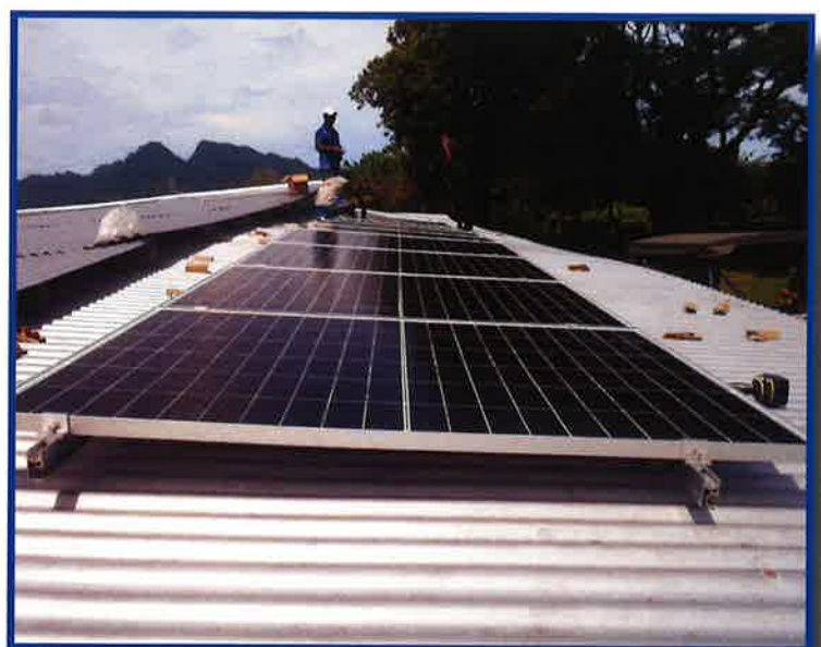
Above: 12 Solar Panels Installed
