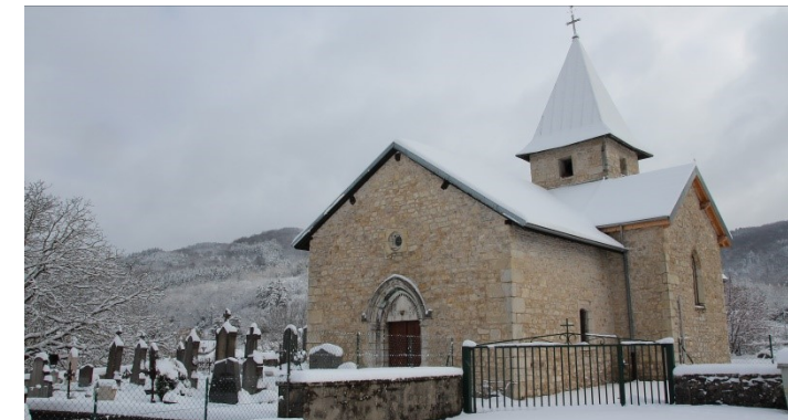
Church of La Balme, site of the first Bugey mission, Jan 1825
